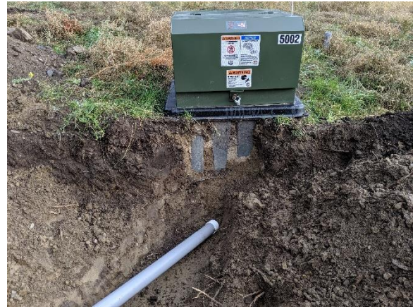
PAD-MOUNTED TRANSFORMER
